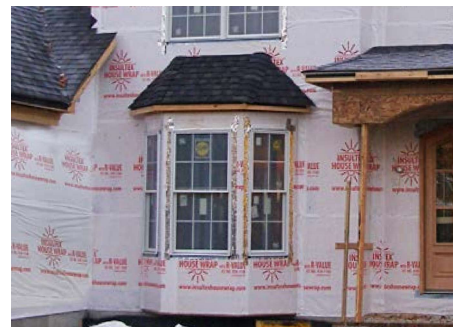
Additional R-6 Insultex House Wrap Insulation on Walls (R-21 standard)
