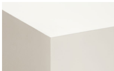
Finished Ceiling Joint
