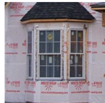
R-6 Insultex House Wrap Insulation on Walls
